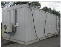
The Main 13.8kv Substation has been designed and built to house a 13.8kv Switchboard, 100kva Transformer and associated equipment. One external equipment & personnel access double door is provided. Fitted internal panic bar release; removable panel above door provided to increase maximum available headroom to 3metres. Access & Stair are provided.
